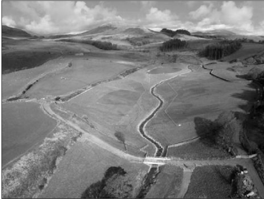
Figure 9. Baystone Bank Reservoir – after
